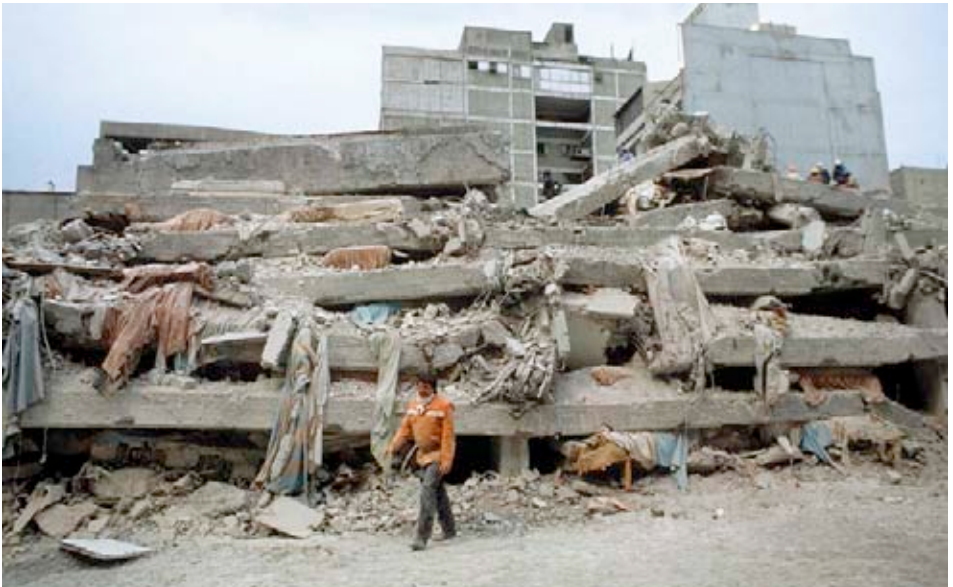
In ruins: an earthquake in Mexico left thousands dead and 20,000 families without shelter.
