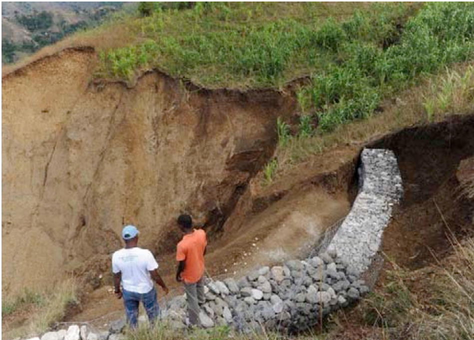
Protection against erosion in Haiti: through a “cash for work” project Diakonie Katastrophenhilfe built stone walls to counteract soil erosion in the mountains of Petit Goave.
