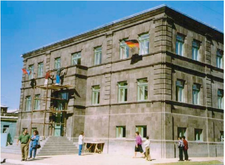
Diakonie Katastrophenhilfe supported the restoration of infrastructure.
