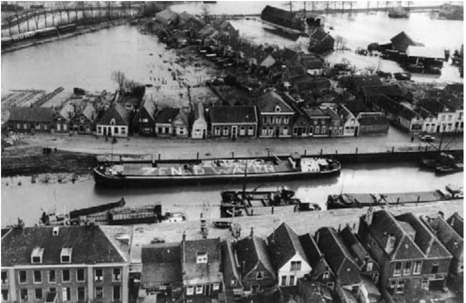
Zend Water (send water) was written on the boat in Brouwershaven in the Netherlands: flood victims were cut off from food and drinking water.
