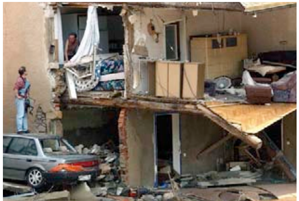
The extent of the damage caused by the flood in 2002 was worse than initially thought.
